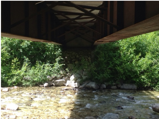
Left Bank Abutment when facing downstream
