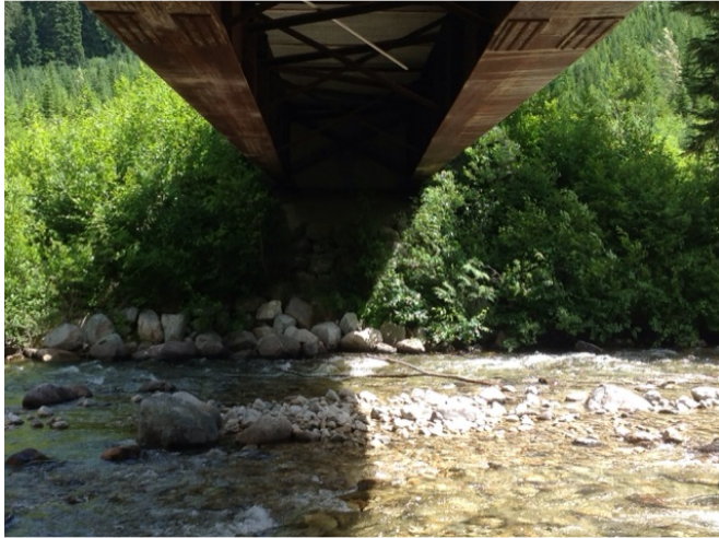
Right Bank Abutment when facing downstream
